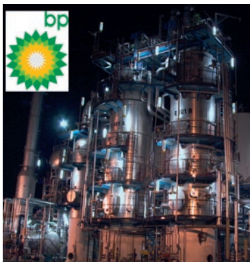
Biturox® Plant, Lavera | France
