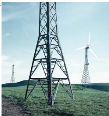
Lattice mast towers for wind energy
