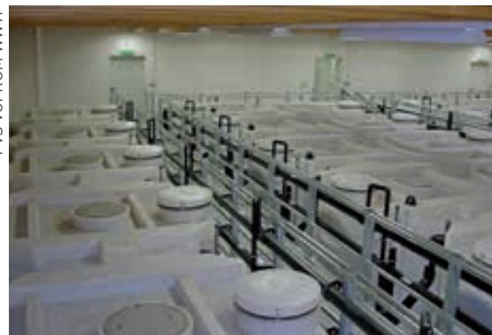
PVS VOPROM WWTP
