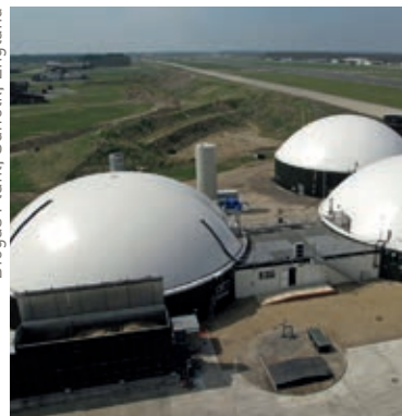
Biogas Plant, Suffolk, England
